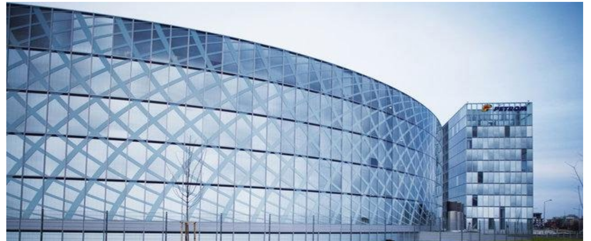
OMV PETROM CITY BUILDING
